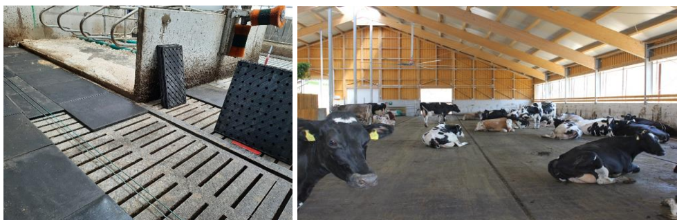
Figure 3. Floor separating urine and faeces (left); artificial permeable floor (right)
